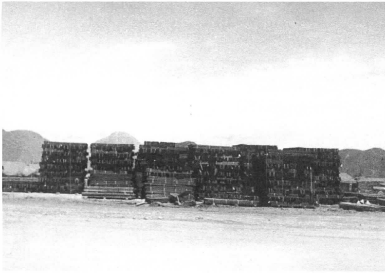
Stacks of steel (PSP) grating used for airstrips and other types of roads, floors, etc. In Qui Nhon
