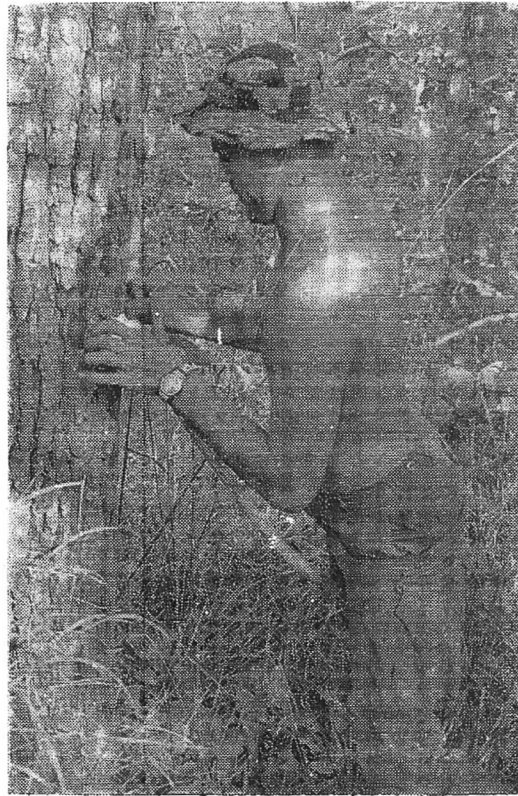
FIRE IN THE HOLE — Preparing to blow a landing zone (LZ) for a MEDEVAC, Private First Class Ronnie G. Woods of Tulsa, Okla., packs plastic explosive at the base of a tree. Woods is assigned to Company A, 326th Engineer Battalion (Airborne).
