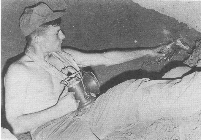
TUY HOA, VIETNAM (101st-IO) -- Private First Class Johnny Vermillion of Grundy, Virginia, a member of the 1st Brigade, 101st Airborne Division's Company "A", 326th Engineers removes punji stakes from the walls of a tunnel complex uncovered by the "Screaming Eagles" near Tuy Hoa.
